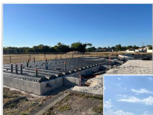
Premiers parpaings, isolation et chappe
